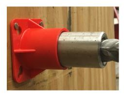
4.Use nail holes to mount FMP to wooden form. Ensure FMP is secured properly to prevent movement prior or during pour.
